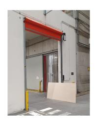
It can be used to separate two temperatures ranging from  $-30^{\circ}$ C to  $+40^{\circ}$ C.
